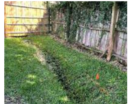
Existing backyard flooding
