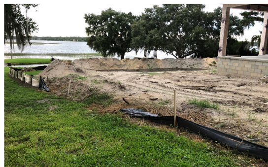
Examples of improperly installed silt fence
