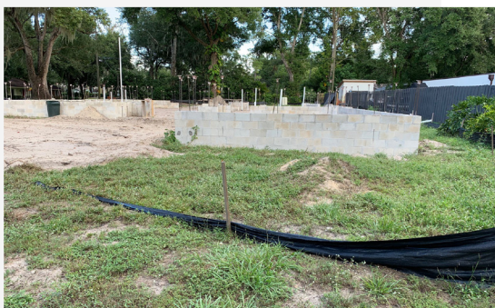
Examples of improperly installed silt fence
