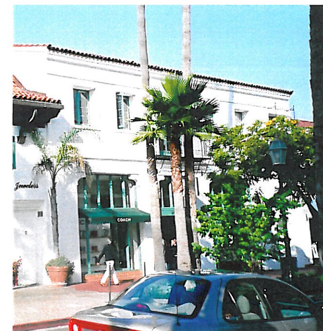
Examples of Main Street buildings showing all the basic storefront façade components: upper façade, expression line, storefront and flat roof
