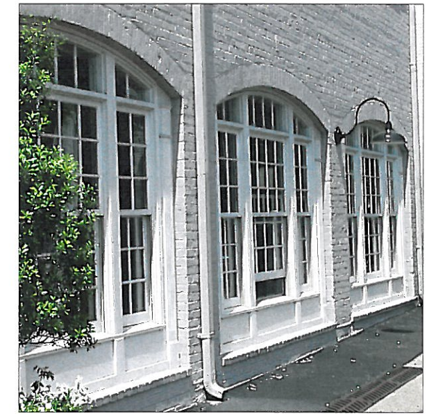
Brick façades with flush arches and projecting brick sills
