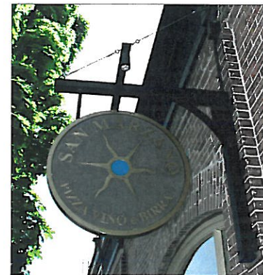
Lighting attached to Sign
