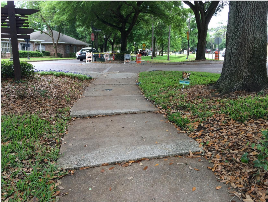
Exhibit 3 – Example of sidewalk joints with tripping hazards
