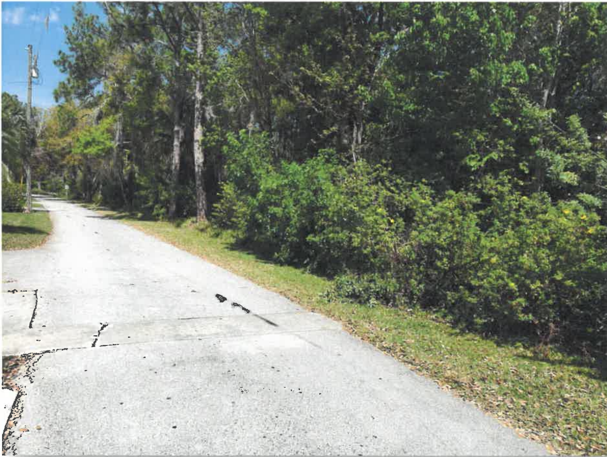
Exhibit 5: Heavily Wooded Portion of Trail, Looking North along S. Lake Butler Boulevard
