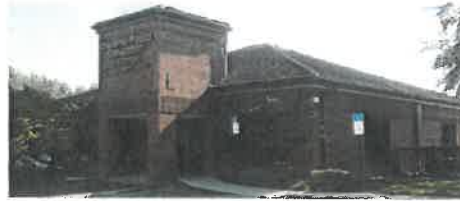
City of Orlando Police Department Metrowest Substation
