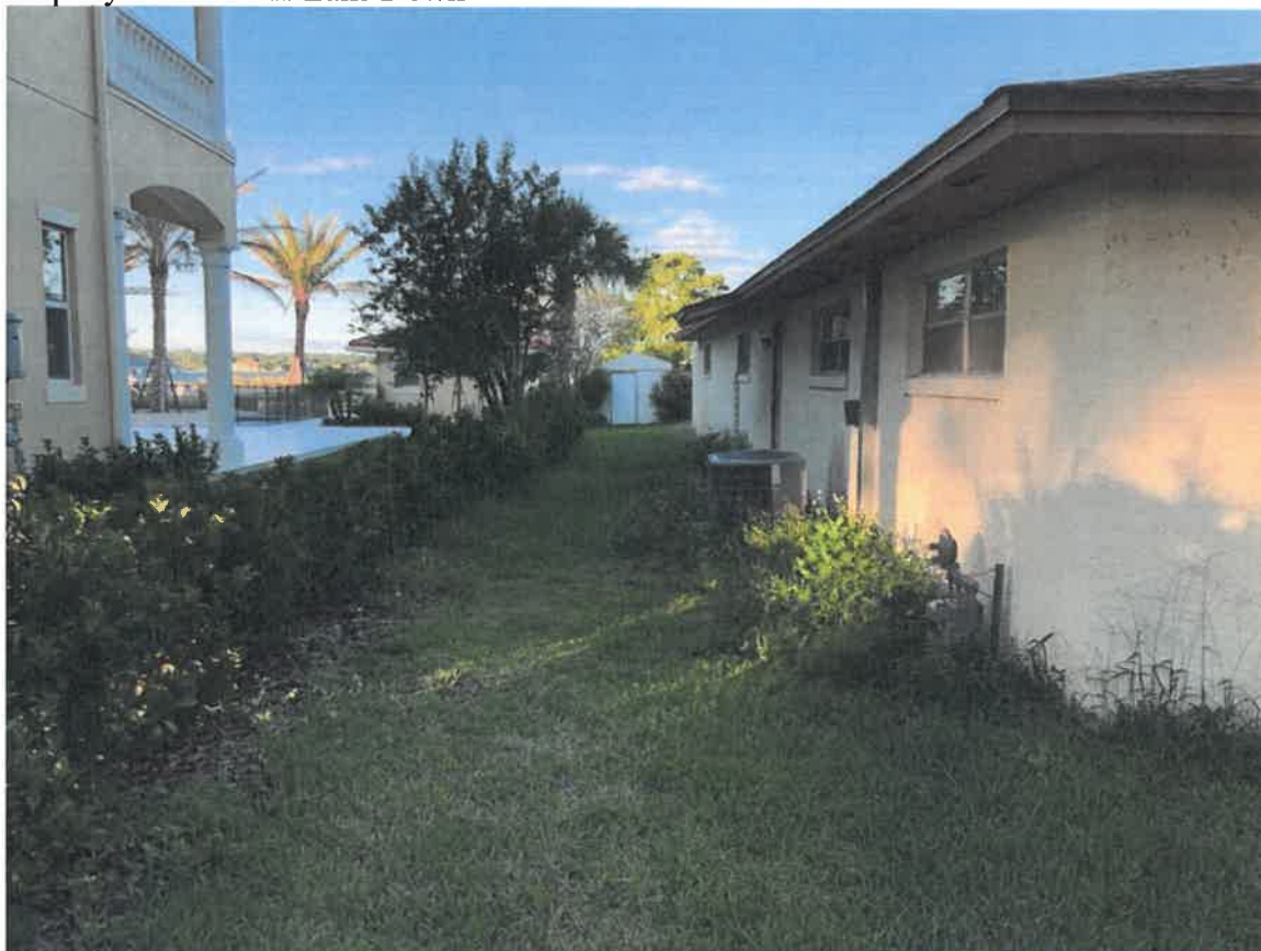
Property line towards Lake Down
