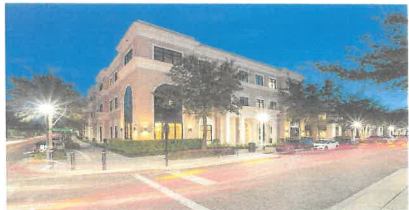
MOTE-MORRIS HOUSE RESTORATION | 07
