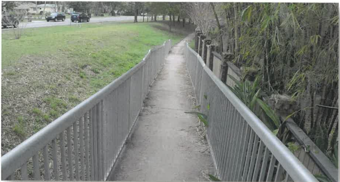
Exhibit 10 – Narrow Path to Existing Pedestrian Bridge
