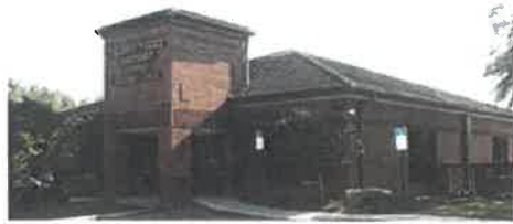
City of Orlando Police Department Metrowest Substation
