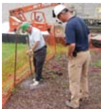
Figure 10. Aeration of soil to relieve compaction in critical root area.
